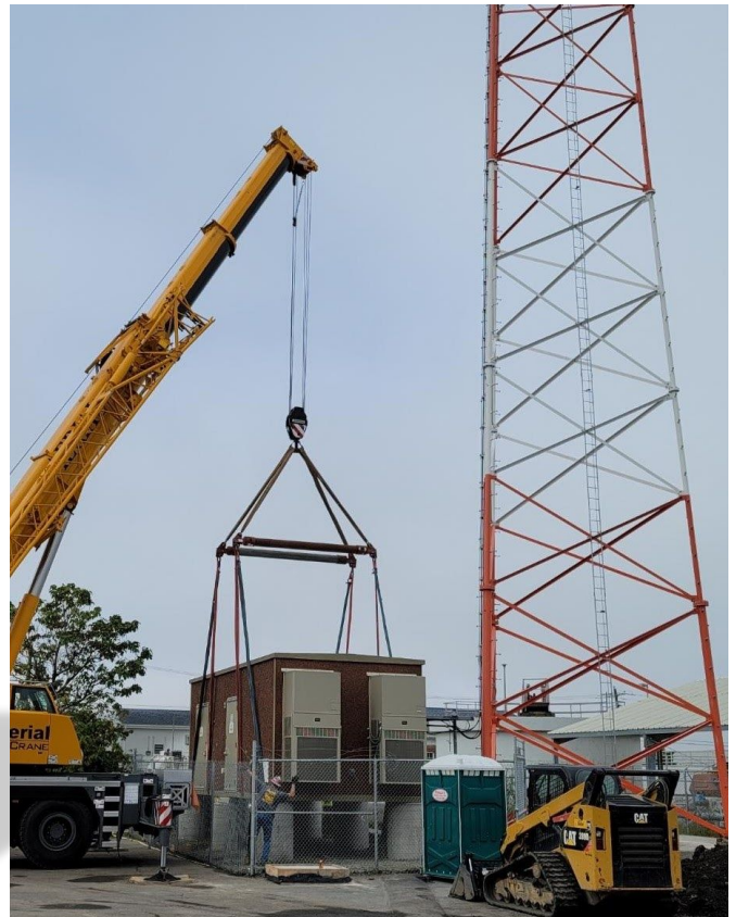
Crisfield, Somerset County shelter installation.
